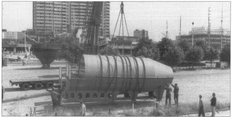
Right: The U-boat section containing the Walter turbine is lowered into position for display at the Deutsches Schiffahrtsmuseum.
