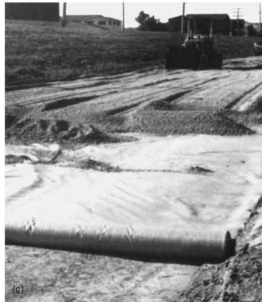
Fig. 1. Geotextiles are used to stabilize soils. (a) A rutted and unstable surface results from subgrade deformation and intermixing between subgrade soil and aggregate base. (b) Geotextiles resist rutting through separation and reinforcement (from Mirafi Fabrics for the Mining Industry, Celanese Fibers Marketing Co. ). (c) A highway base course constructed with geotextile between subgrade and aggregate base (from Mirafi Family of Construction Fabrics/MPB8, Celanese Fibers Marketing Co. ).
