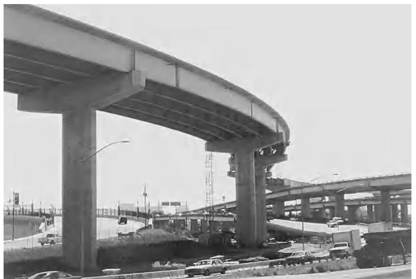
Fig. 2. Steel girder bridge.
