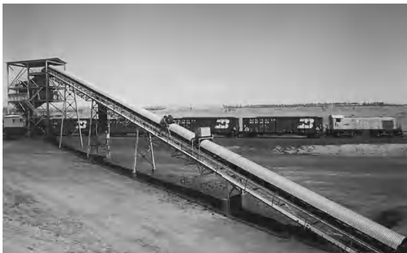
Fig. 19. Hopper cars being loaded by a belt conveyor. (Burlington Northern, Inc.)
