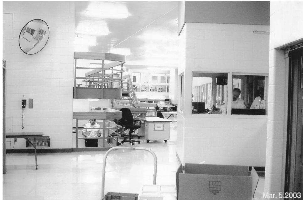
Photo 1 View of the control station and half of the unit
