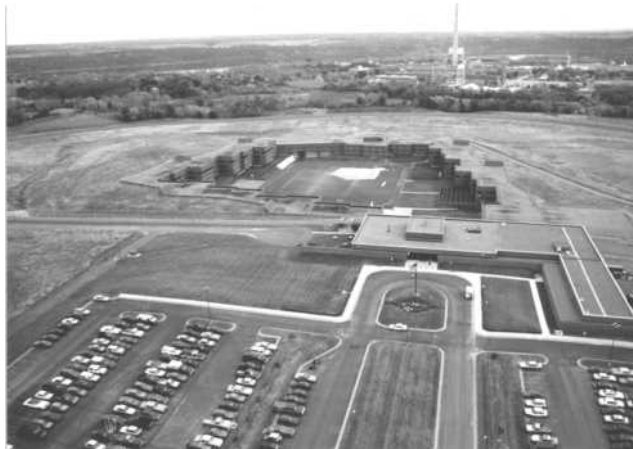
Photo 1 Oak Park Heights, administrative building in the foreground
