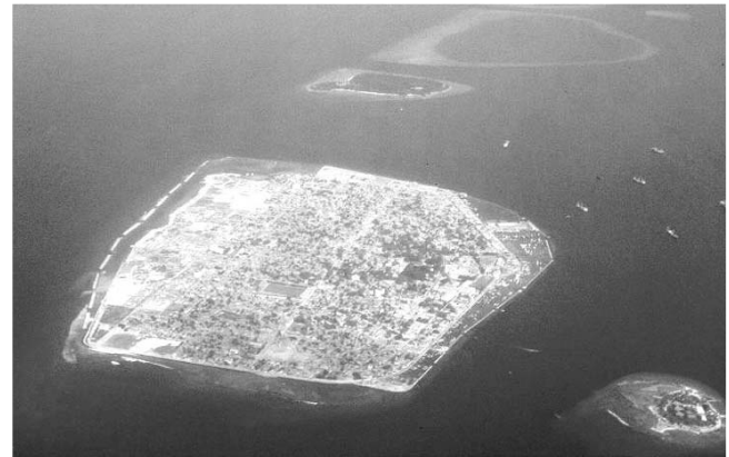
Figure C74 The capital city and island of Malé, Republic of Maldives; a coral reef island city. The reef flat is almost entirely infilled. A break-water (on left) was built by Japanese aid following devastating surges and loss of land. Water abstraction has left the water table damaged, now with saline and sulfurous water.
