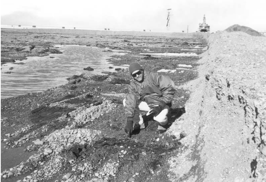
Figure W32 Bill Streever points to peat exposed by removing gravel from an abandoned work pad near the Beaufort Sea on the North Slope of Alaska. Gravel removal is the first step in tundra rehabilitation.
