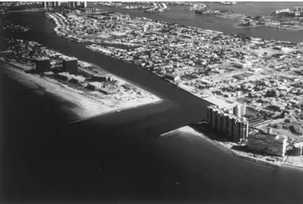
Figure H14 Jetty at a tidal inlet showing a significant amount of downdrift erosion as the result of the inability of sediment to cross the structure and the inlet.
