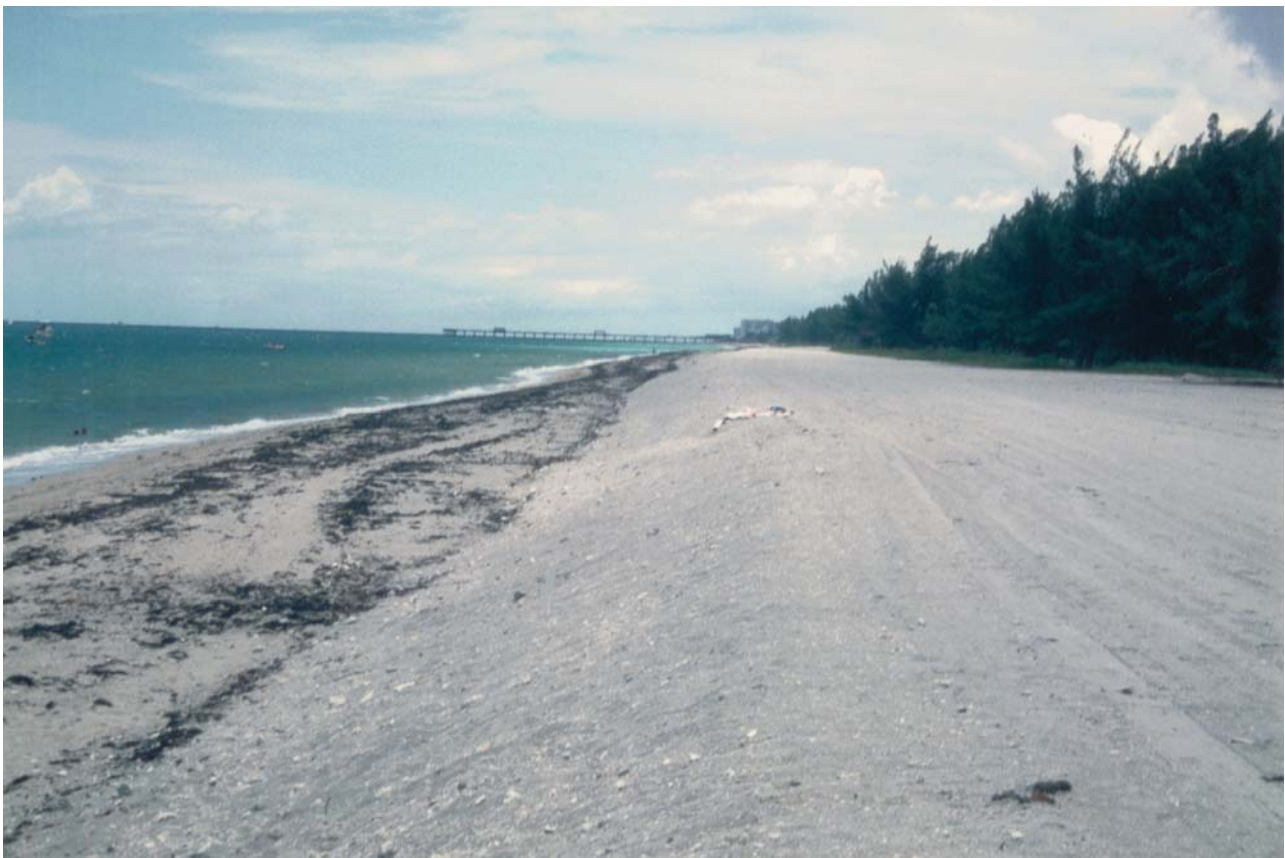
Figure B31 Example of a large beach-replenishment project involving more than 6 million m 3 of sand that was pumped from offshore in south-east Florida near Port Everglades (Fort Lauderdale). As shown in the photo, the beachfill has been eroded back to the native sand beach (left) and the built beach is perched about 2 m above the eroded beach. The beach scarp that developed during erosion of the fill was graded by dragging a heavy I-beam across the sand. The more gradual slope facilitated access to the water by reducing the hazardous vertical face of the scarp.
