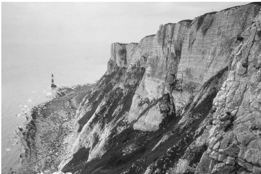
Figure M25 Clifed landscapes require oblique photography to show features, the chalk cliffs of Beachy Head, southern England (original photograph JPD).
