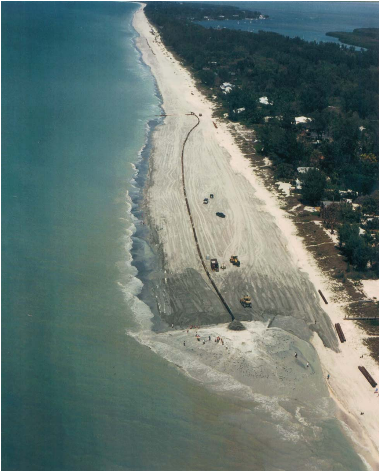
Figure B30 Restoration of Captiva Beach in 1996 on Sanibel Island, southwestern Florida, showing beach-quality sand pumped from offshore via a submerged pipeline to the shore. The sand–water slurry debauches from the pipe end (lower center foreground) to form an alluvial fan that builds up along the shore. Shell hunters often congregate about the proximal part of the sediment fan hoping to find collector's specimens. Shore birds search the distal portions of the fan for crustaceans brought up from the seafloor in the offshore borrow area. Road graders and bulldozers redistribute the pumped sediment into the beachfill design shape that often incorporates overfill that will be sacrificed to the littoral system as the beach equilibrates to the ambient wave climate. The beachfill is sometimes initially somewhat darker than the native beach sand, as shown here, due to a small percentage of organic content. Organic matter in the fill bleaches out within a few weeks and the native-colored sands imperceptibly grade into the fill material. Pipe extensions lie at the foot of the foredunes (photo, lower right) and mark the approximate position of the back berm (photo: Courtesy of Coastal Planning and Engineering, Inc., Boca Raton, FL).
