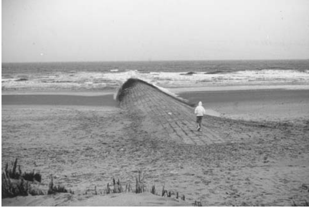
Figure H13 Large groin on the North Sea coast where there is little difference in accumulation of beach sand on either side of the structure.
