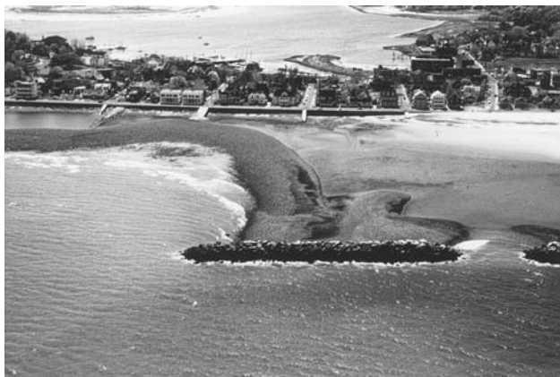
Figure H15 Photograph of a detached breakwater designed to protect the shore landward of it. (Courtesy of D. FitzGerald.)
