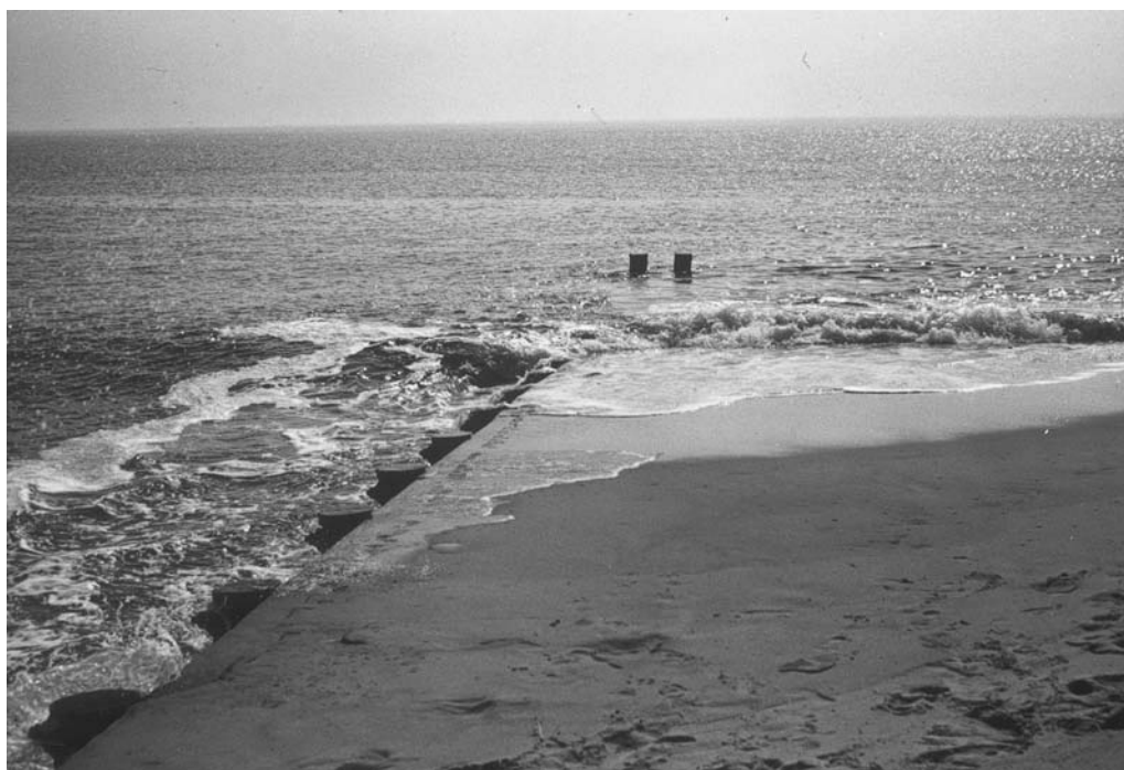
Figure H12 Groin showing a significant amount accumulation on the updrift side.
