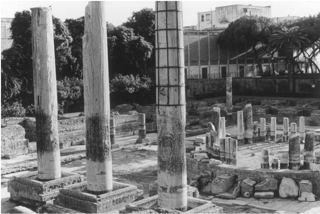
Figure T3 The “Temple of Serapis” in Pozzuoli (Italy). Note the dark band on the columns produced by molluscan borings (the upper limit of which is slightly less than 6 m above the paving of the “Temple,” which is partly flooded by a few centimeters of water) (Photo D388, October 1991). The same floor appears more submerged in photos taken in 1982–83 (Vita-Finzi, 1986, p. 10).
