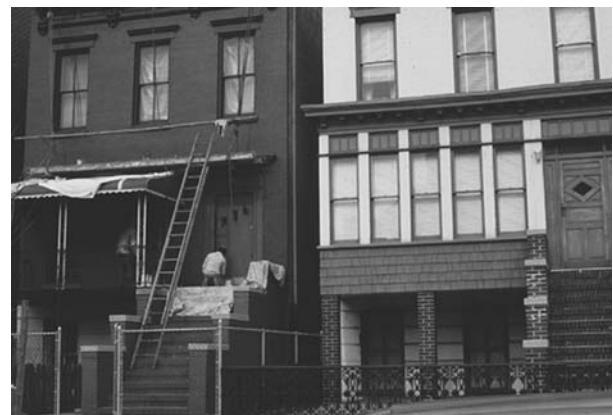
Figure 1 Example of Intracultural Diversity in Terms of Housing in the Neighborhood
