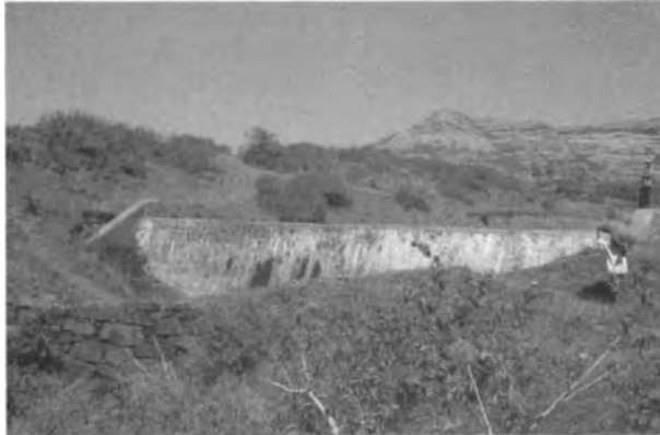
Fig.R.3: Check dams act as water reservoirs, where water can be used for irrigation purpose. Courtesy: Dr. Vrishali Deosthali, Department of Geology, University of Pune, India.
