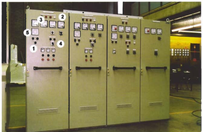
A synchronising panel showing: 1. Circuit breaker closing pushbuttons 4. Speed control generator 2. Voltmeter busbar-generator 5. Synchronoscope 3. KW indicator 6. Main circuit breaker 7. Synchronising equipment
