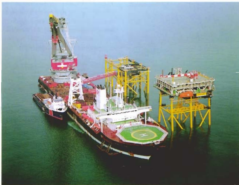
Crane vessel installing fixed platform
