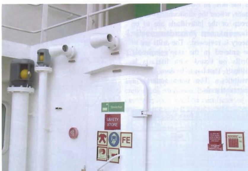
Entrance door with name and technical marking
