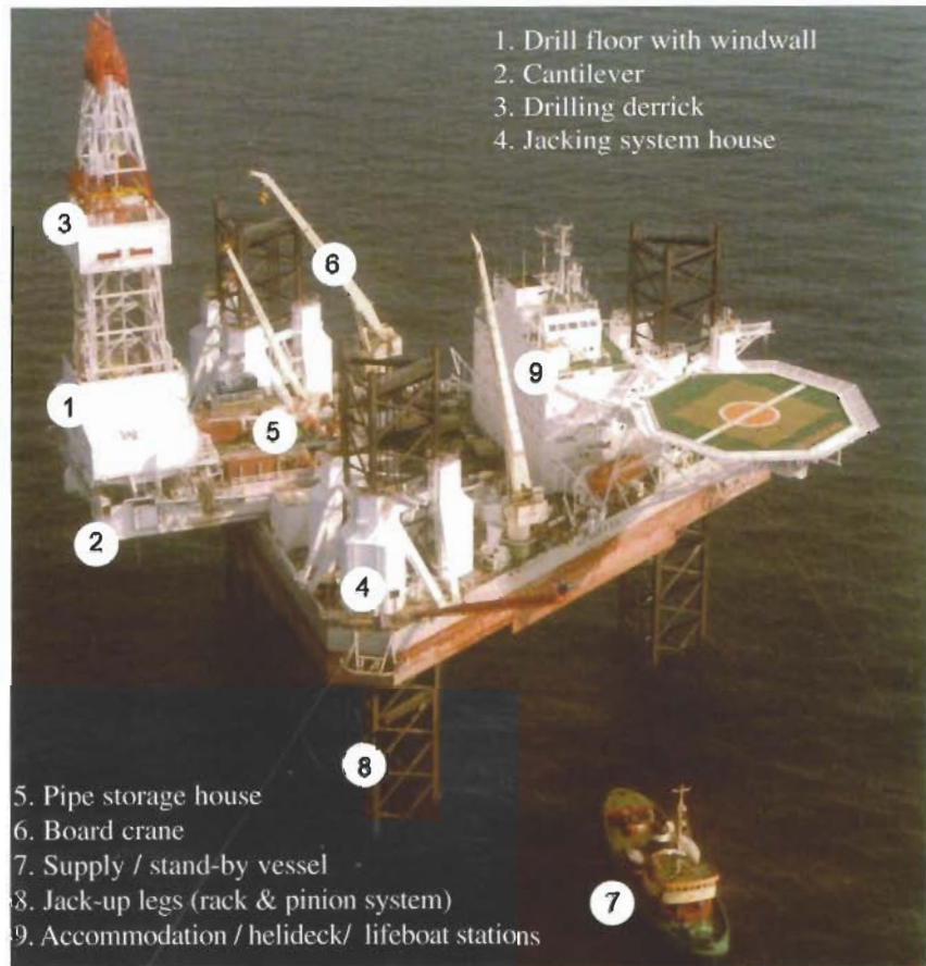
Jack-up rig in drilling mode, suitable for arctic conditions
