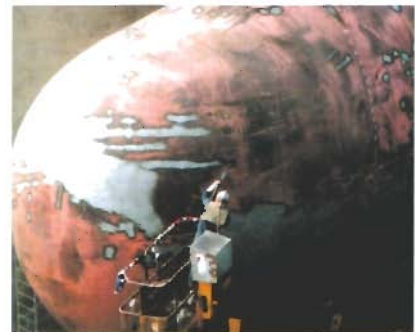
The old paint-layer is removed by gritblasting
