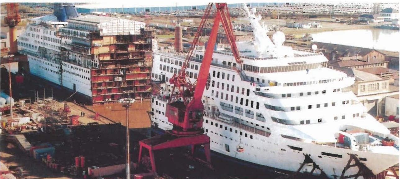
A passenger ship is being lengthened to increase capacity.
