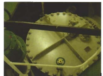
Water inlet filter
