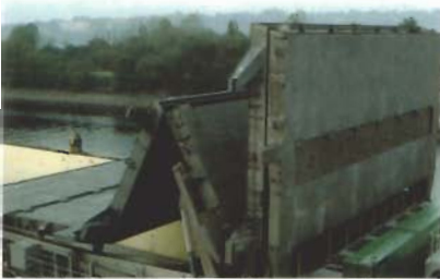
Folding hatch with cylinders on the outside
