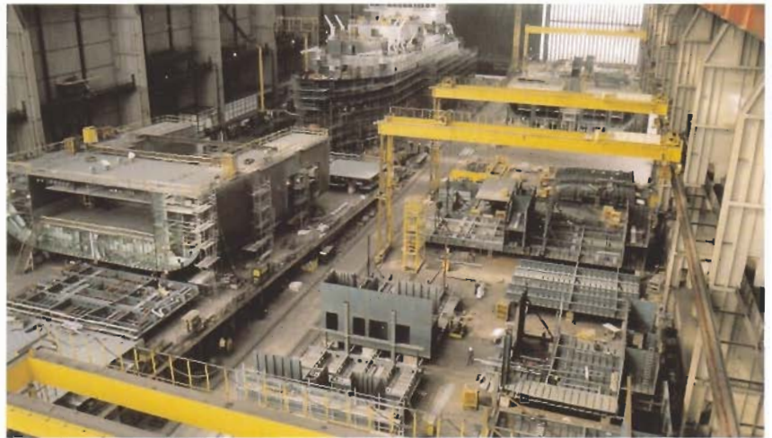
View in an assembly shop
