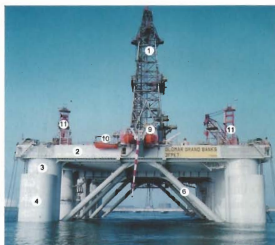
semi submersible at operational draught
