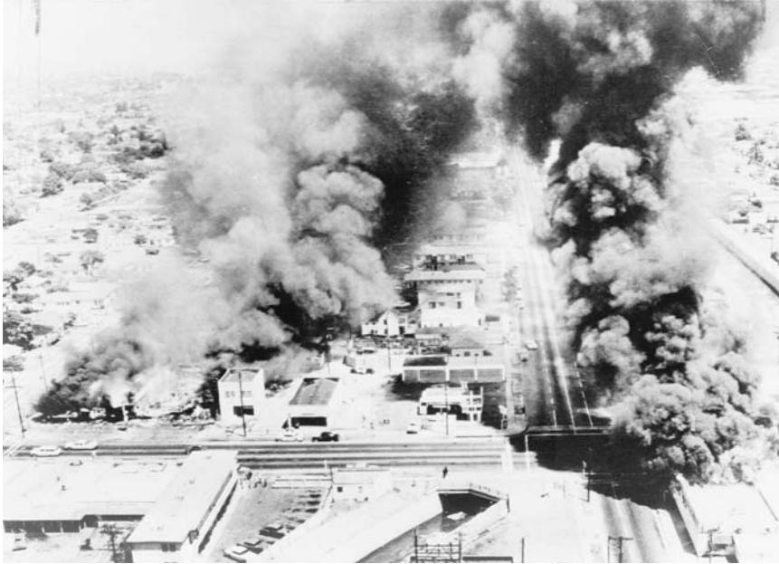
Buildings burn during the Watts riot in Los Angeles, August 1965. (Library of Congress)
