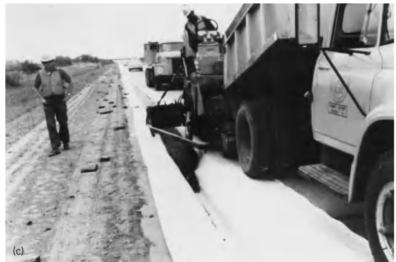
Fig. 2. Geotextiles find wide use for drainage. (a) Without a filter, soil particles may wash into and clog the drain. (b) Drainage fabric provides retention at the soil-drain interface, while allowing water to pass through (from Mirafi Fabrics for the Mining Industry, Celanese Fibers Marketing Co. ). (c) Drain trench lined with a geotextile and backfilled with coarse aggregate.
