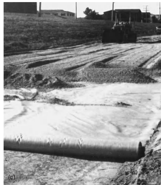
Fig. 1. Geotextiles are used to stabilize soils. (a) A rutted and unstable surface results from subgrade deformation and intermixing between subgrade soil and aggregate base. (b) Geotextiles resist rutting through separation and reinforcement (from Mirafi Fabrics for the Mining Industry, Celanese Fibers Marketing Co. ). (c) A highway base course constructed with geotextile between subgrade and aggregate base (from Mirafi Family of Construction Fabrics/MPB8, Celanese Fibers Marketing Co. ).
