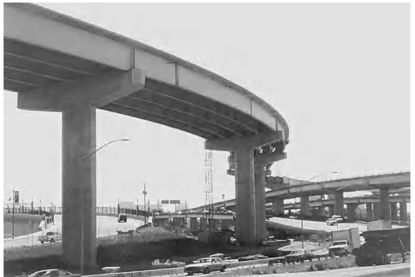
Fig. 2. Steel girder bridge.
