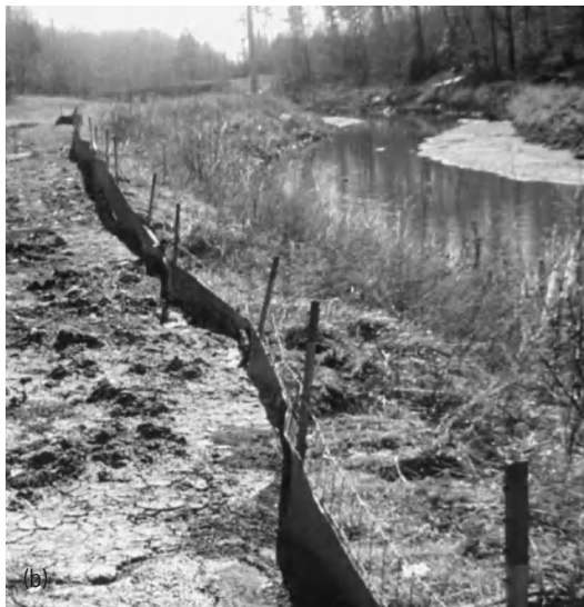
Fig. 3. A silt fence is a fabric-lined fence structure. When lined with a geotextile, it retains sediment runoff, preventing contamination of adjacent waterways. (Mirafi Fabrics for the Mining Industry, Celanese Fibers Marketing Co.)
