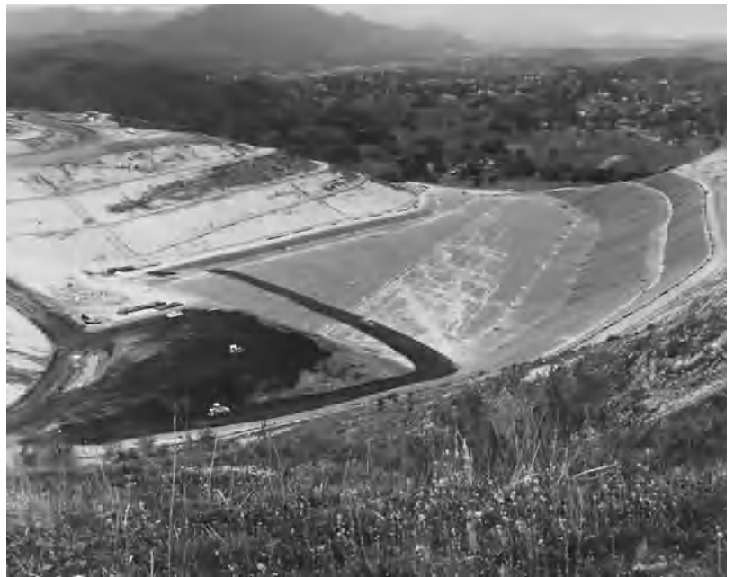
Fig. 4. Calabasas solid-waste landfill in Los Angeles County, California, being lined with geomembrane.
