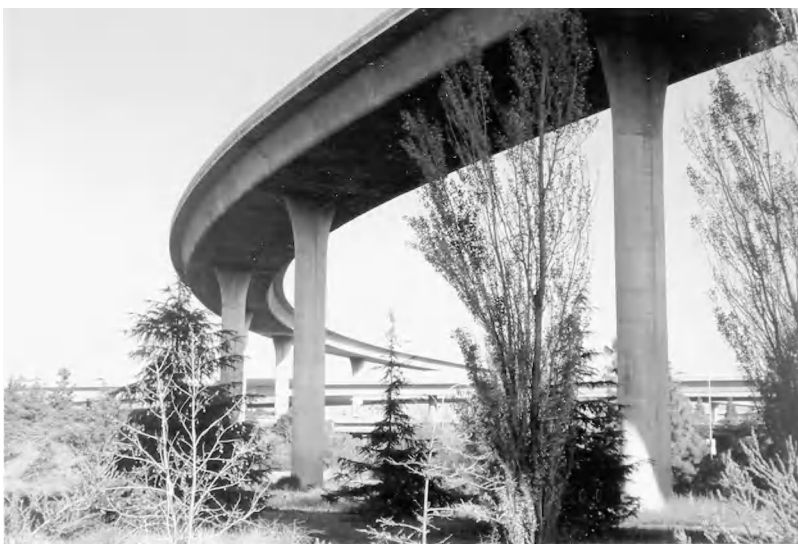
Fig. 3. Concrete girder bridge.
