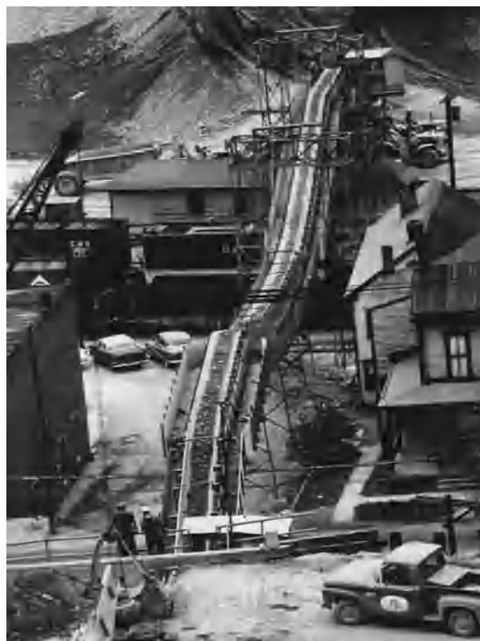
Fig. 2. Conveyor carrying rock over a railroad yard.
