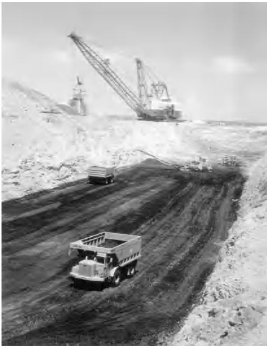
Fig. 6. Dragline working from the surface of the ground. (Morrison Knudsen Co.)
