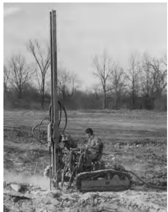
Fig. 7. Crawler-mounted drill. (Gardner-Denver)
