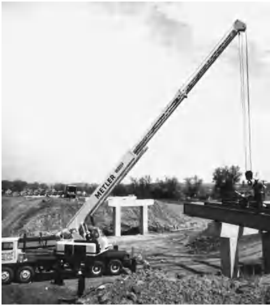
Fig. 1. Hydraulic truck crane.
