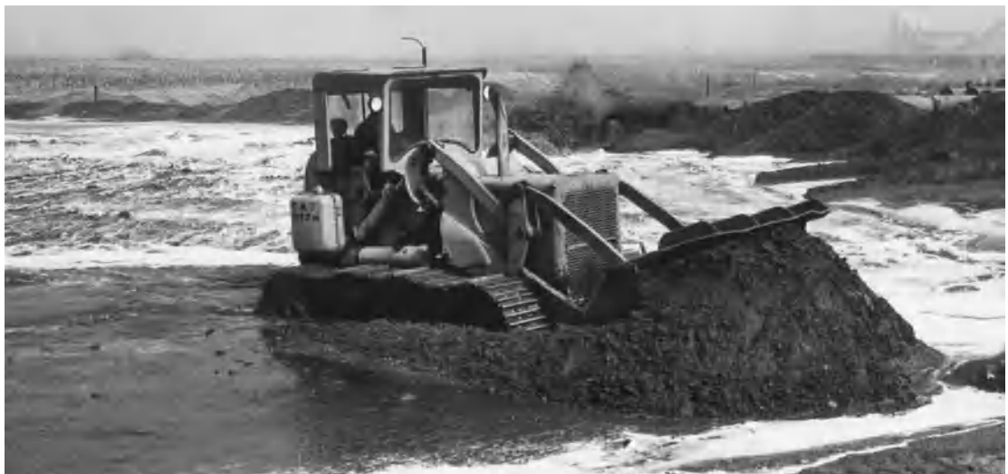
Fig. 4. A loader operating in a swamp.
