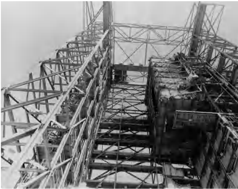
Fig. 4. Upper part of a Titan 3 service structure showing the enclosure which provides shelter for the payload. (TRW Systems)
