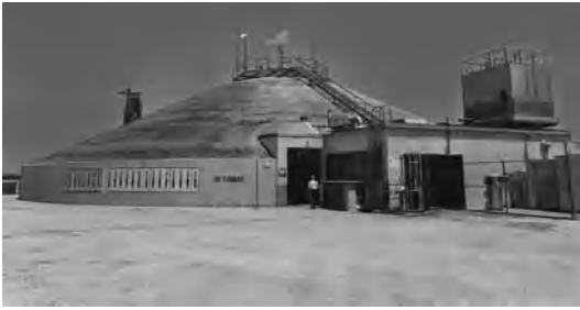
Fig. 6. External view of typical blockhouse for uncrewed missions. Massive concrete construction protects workers during launch.
