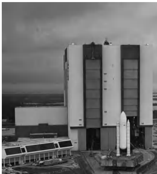
Fig. 8. Space shuttle Vehicle Assembly Building on Complex 39 at the Kennedy Space Center. The launch control center is at lower left. The space shuttle is on the mobile launch platform in front of the building. (NASA)
