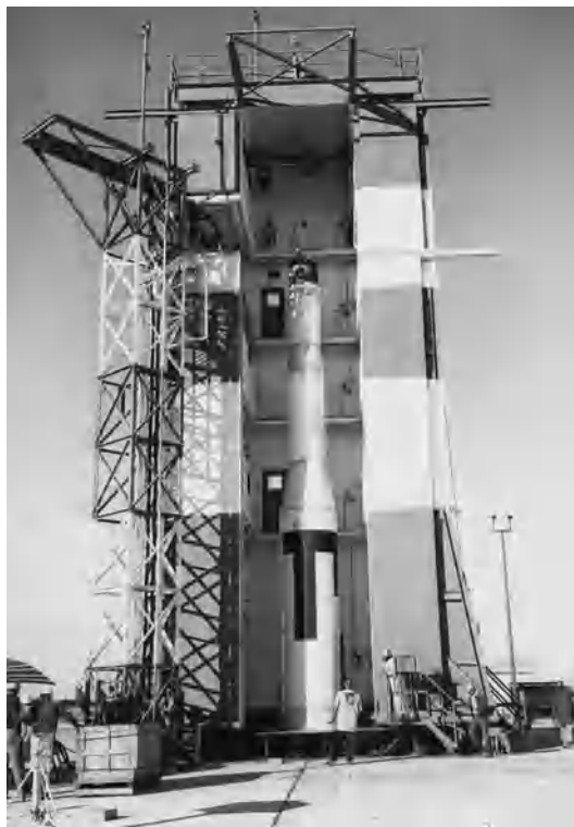
Fig. 3. Minuteman ICBM on the launch pad with its service structure in place. (Boeing Aircraft)
