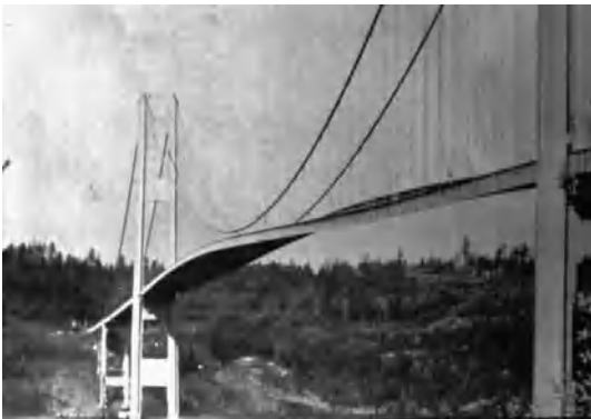
Fig. 3. Tacoma Narrows Bridge in the middle of its wild oscillations, a little before it collapsed.
