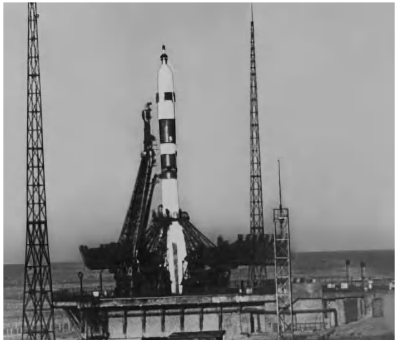
Fig. 2. Launch pad with Soyuz spacecraft and rocket. Gantry and hold-down mechanisms fold back at proper moments in launch sequence. (Tass, from Sovfoto)
