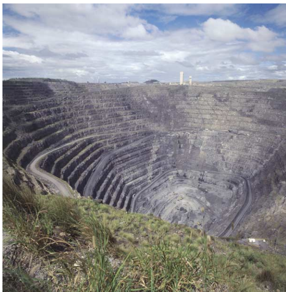
Figure 6 Palabora mine open pit, averages 1750 M across the rim and has reached its economic working depth of 822 M in 38 years. Beneath the open pit underground mass mining by block caving methods is now producing 30 000 tonnes per day of copper ore from the core of this very productive carbonatite pipe. Photograph courtesy of Rio Tinto plc.
