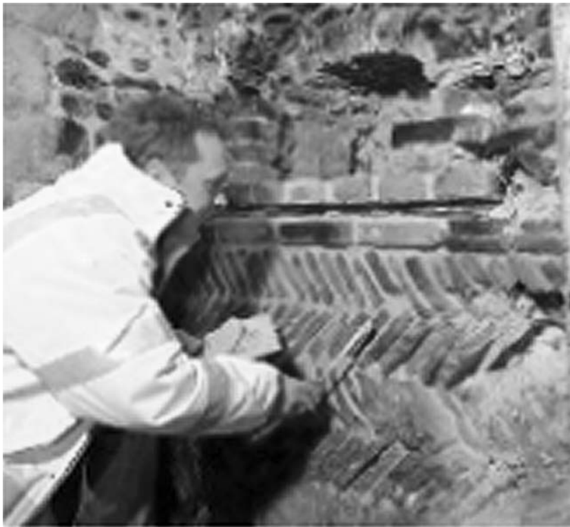
Fig. 2 Uncovered medieval fireplace (Courtesy of Chichester District Council, England).
