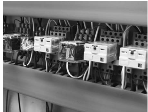
Fig. 1 Relay logic to cycle certain zones, temporarily, with timed-out latch release.
