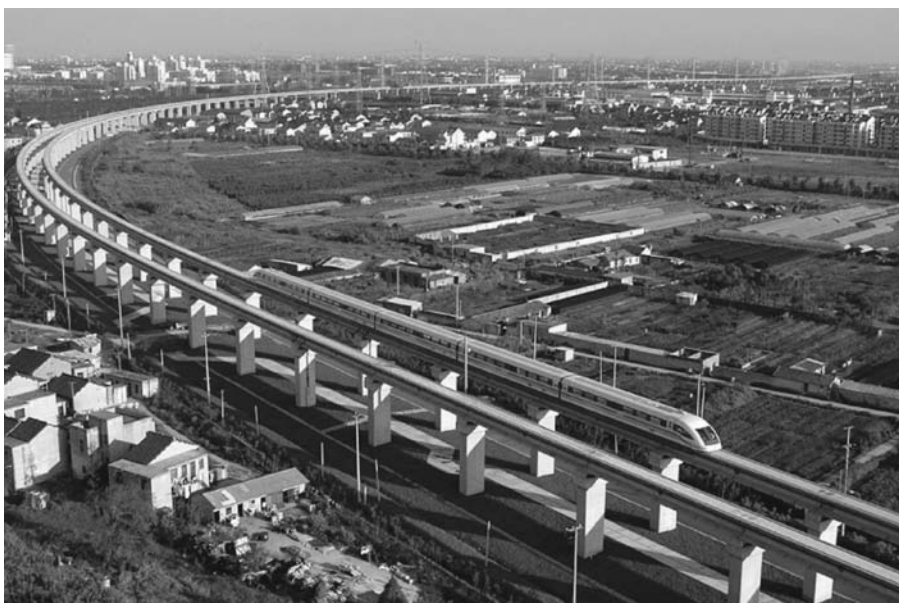
Fig. 3 Elevated 267 mph Shanghai Maglev is on time 99.9% of the time and places a minimal footprint on the landscape and does not cut communities in half or obstruct their existing road networks. Photo courtesy of Transrapid International.
