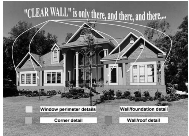
Fig. 3 Framing lies behind a significant portion of the wall area in many houses. Source: From ASHRAE Special Publications (see Ref. 9).
