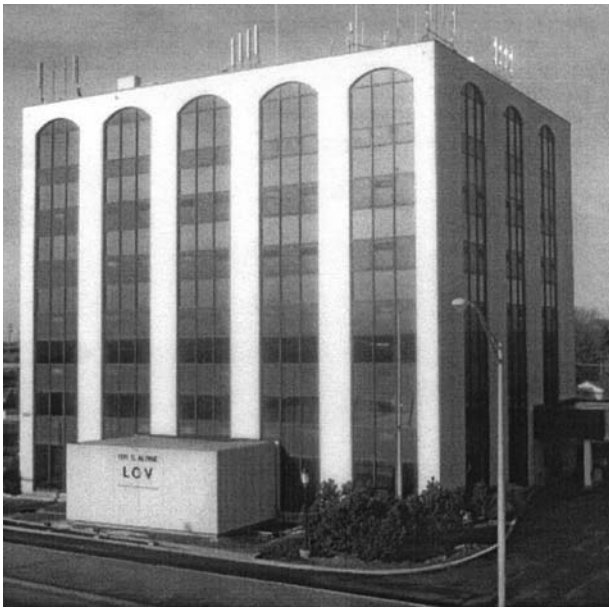
Fig. 1 Demonstration building following film installation.
