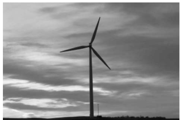
Fig. 5 Projects and technologies should be appropriate and meet needs, which may call for innovative and creative approaches. There are great renewable energy resources on Tribal lands, but their development sometimes requires different thinking about organizational structure, financing, management, and training.
