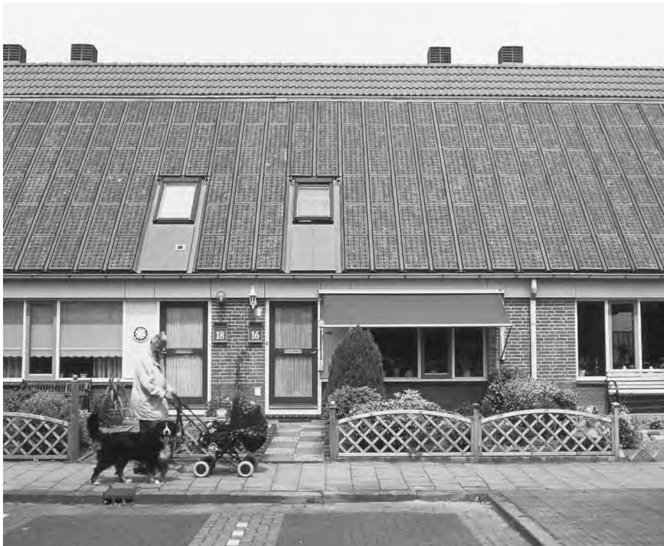
Array of solar panels (photovoltaic cells) on the roof of terraced houses in Heerhugowaard in the Netherlands. This is part of a Dutch government pilot project to investigate clean, renewable energy forms such as solar power. The 10 houses in this terrace (only two seen here) have a total of 200 square meters of solar panels on their roofs. The total power output of these solar panels is 24.6 kilowatts. The photovoltaic cells contain a semiconducting material that converts sunlight directly into electricity. Solar power is relatively cheap, as once the panels are installed, they continue to produce electricity indefinitely. (Courtesy of Martin Bond/Science Photo Library)
