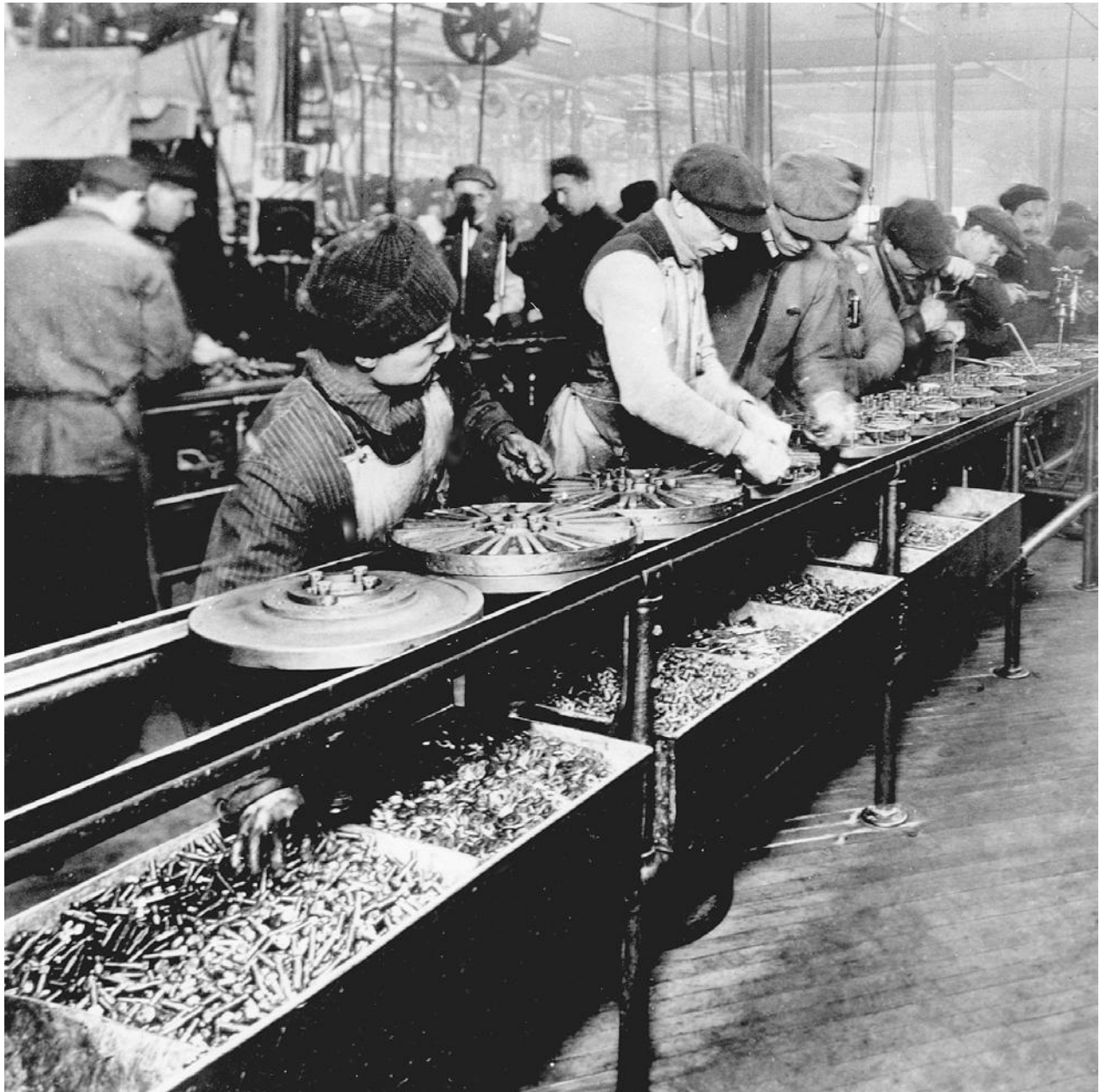
Flywheel assembly line at the Ford Motor Company's Highland Park, Michigan, plant ca. 1913. ASSOCIATED PRESS, FORD MOTOR COMPANY
