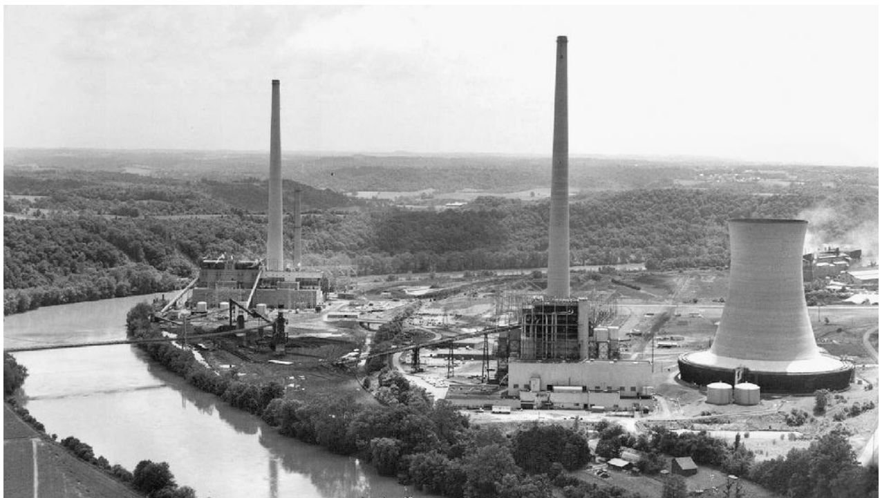
American Electric Power's Muskingum River Plant, Beverly, Ohio, was named in an Environmental Protection Agency lawsuit in 1989. AP IMAGES
