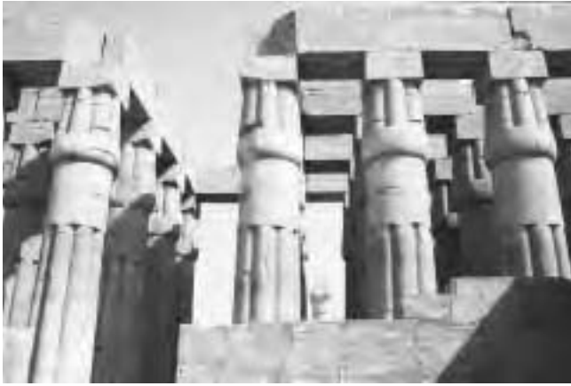
Hypostyle columns displayed in the temple of Luxor in the papyrus bundle design. (Courtesy Steve Beikirch.)
