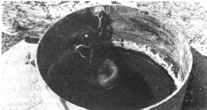
Float-valve regulates water level in stock tank.
