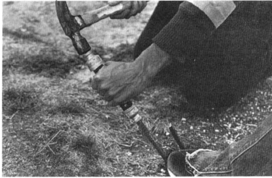
Place the driver over the sharpened end of the rebar stake and hammer it in.
