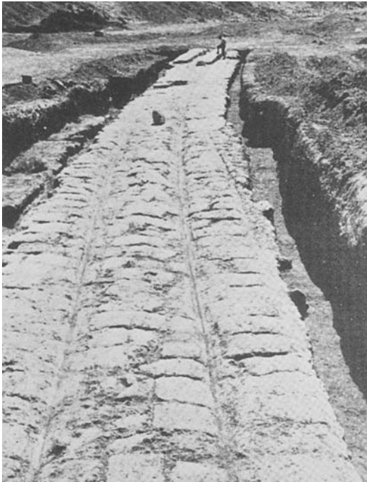
diolkos View of the diolkos , the stone haulway across the isthmus of Corinth probably built c.600 BC. Its chief aim was probably to levy dues on *trade, especially the long-distance seaborne commerce between the Aegean and Italy and the west. From Ralf Krumeich, 'Porträts und Historienbilder der klassischen Zeit', in AM 71 (1956) 209–240, fig. 5. © WBG Darmstadt.
