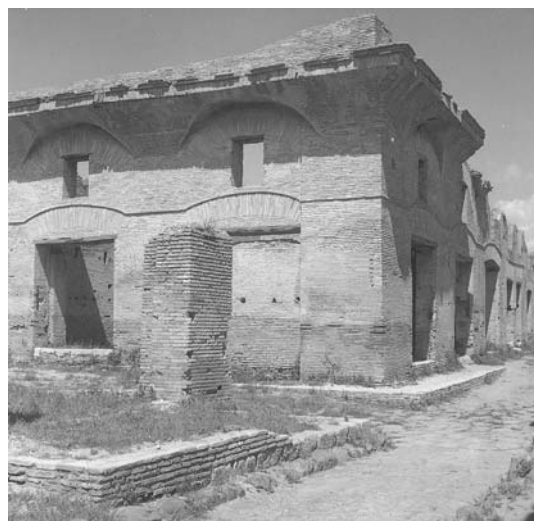
Ostia The brick-faced House of Diana at Ostia (c. AD 150), originally with at least four floors, is a good example of the multi-storeyed apartment blocks ( insulae ) found in the Roman empire's larger cities. In Italy, the use of fired brick (mid-1st cent. AD on) in place of timber-framed mudbrick made this type of structure much safer. Fototeca dell'Unione Internazionale, American Academy in Rome
