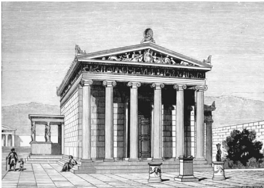
A reconstruction of the east face of the Erechtheum shows its sculpted frieze (the band located directly above the columns) and an outdoor altar. NORTH WIND PICTURE ARCHIVES
